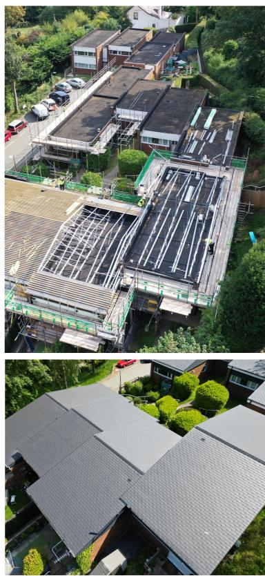
Conducting a thorough structural assessment of the existing flat roof to ensure compatibility and feasibility of the Britframe required careful analysis and engineering expertise. Coordinating the installation of the Britframe and Liteslate with existing roof features, such as skylights or ventilation systems, posed challenges in achieving a seamless integration.
