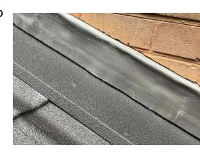
7 Seal the Scribed Area: Apply silicone sealant in a matching colour to the scribed area to ensure a watertight seal.
