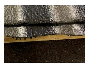
**Note:** The size of the vent strip depends on the roof pitch: use a 10mm strip for pitches of 16° or more, and a 25mm strip for pitches of 15° or less.
