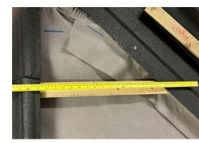
2 Cut the Sheets: Cut the sheets along the marked lines using a nibbler or jigsaw.
