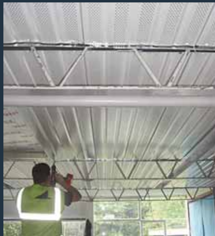
Structural ceiling system
