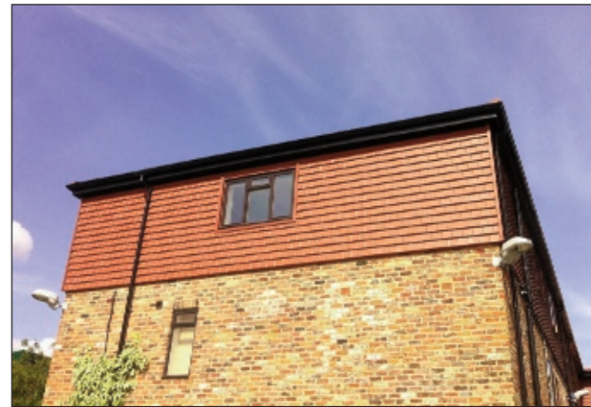
The plain tile's aesthetic characteristics and lightweight properties enable it to be used on a wide variety of applications, including vertical cladding.
