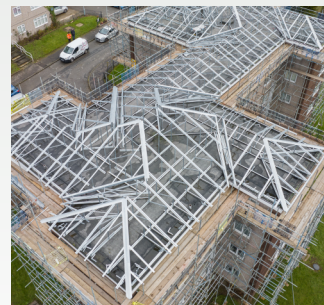
BritFrame Flat-to-Pitch Roof Conversion System
