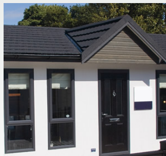
Paint Stipple and Masonry Paint
